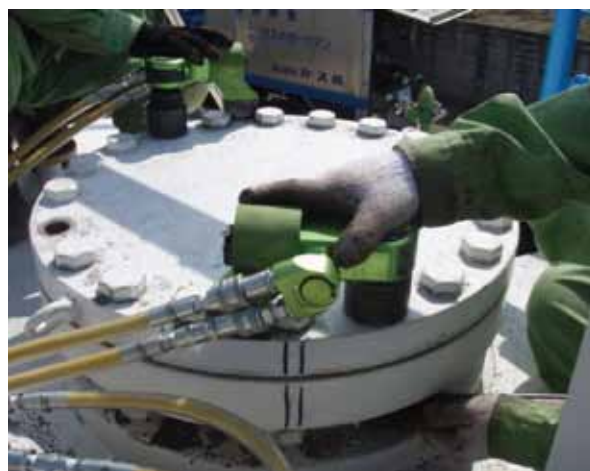
Figure2 Parallel fastening using two hydraulic torque wrenches
