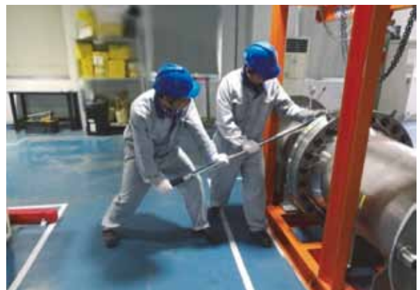
Figure2 Image of tightening
