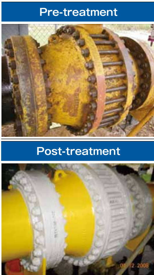
Figure5 A case of rust-proofing treatment
