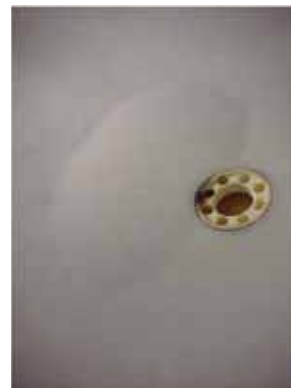
Figure16 Lining around the liquid collection cup is detached
