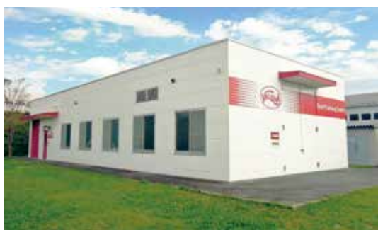
Figure1 Outside view of the VALQUA Seal Training Center™ (Nara)
